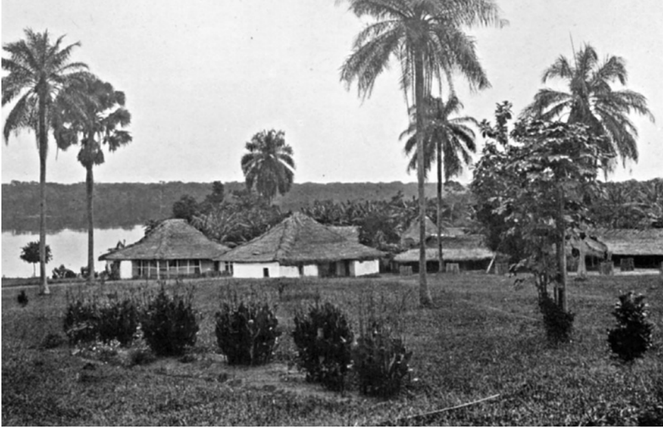
The final decision on Danielsen was taken at the mission station in Ikau.
